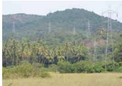
Solution deployment in dense forest 110 kV line, TAN TRANSCO
