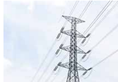
Live line installation 220 kV line, GETCO
